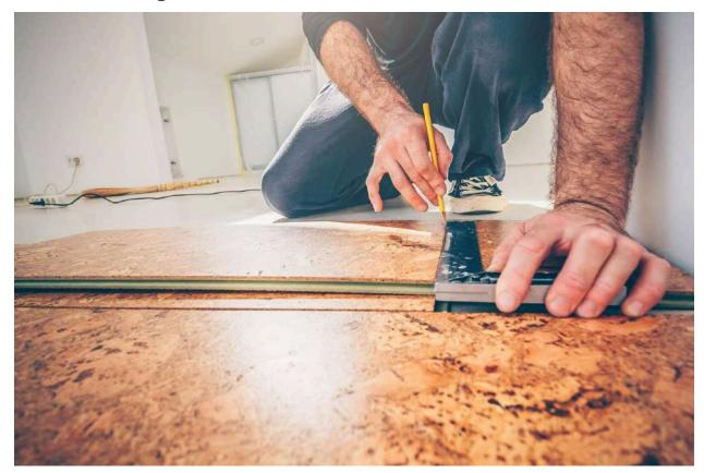
Cork is harvested from the bark of cork oak trees, which regenerate every few years, making it a renewable resource. Cork flooring is soft, hypoallergenic, and resistant to mold and mildew. It provides excellent insulation for sound and temperature, making it energy-efficient. Its natural texture adds warmth to interiors, making it a favorite for eco-conscious homeowners.
