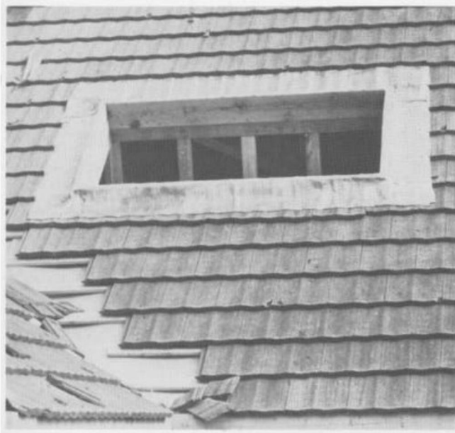
Rooftop skylight openings on many residential homes are edge-flashed with sheet lead for waterproof, weathertight seals. Lead's natural pliability allows it to conform exactly to surface configurations, and also makes it easy to cut, shape, and install the sheet.
