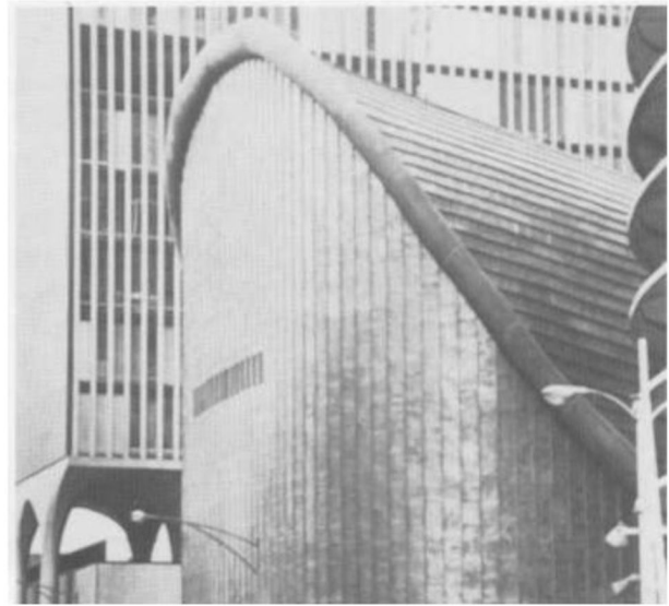
ROOFING AND FLASHING
